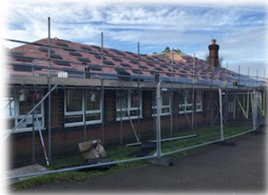
The roof is nearly finished – no more leaks!
